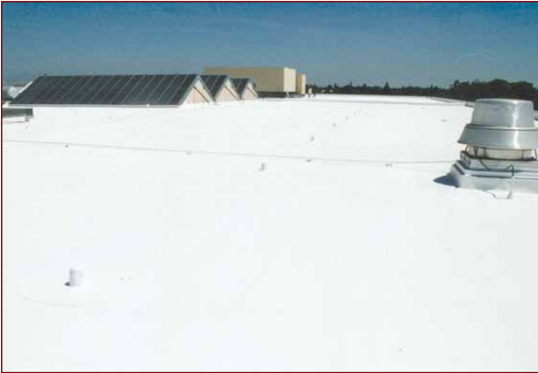
White coatings can provide reflectivity of 70 percent or more.
